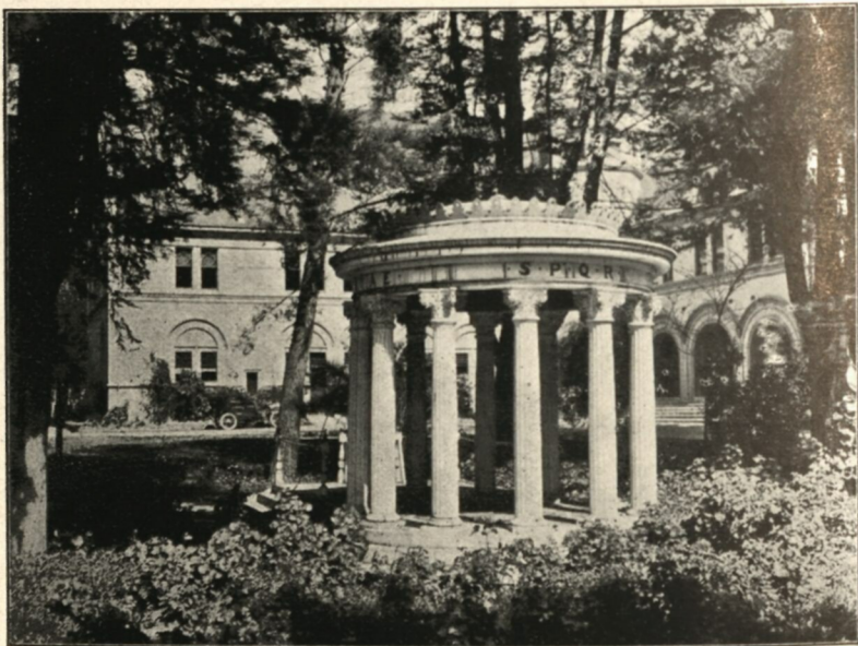
VIEW FROM WEST ENTRANCE OF CAMPUS.
