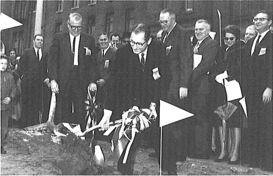
John Tocchini, with shovel in hand, breaks ground on the dental school's new Pacific Heights campus.
